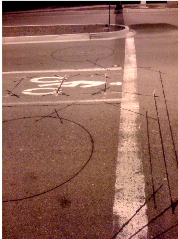
Figure 8: An example of an induction loop, installed beneath a road (making it harder to detect when it breaks!).
